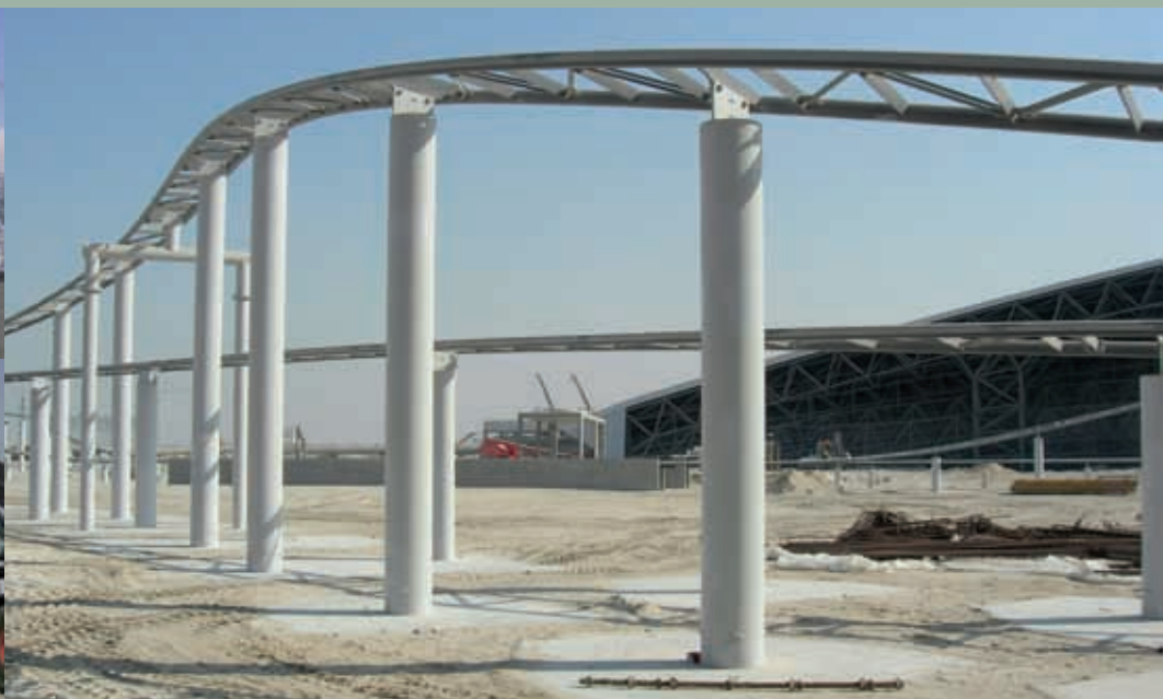
↑ Dueling Coaster, Yas Island, Abu Dhabi • (Erection of 800 tons steel structure, including control and power cable installation)
