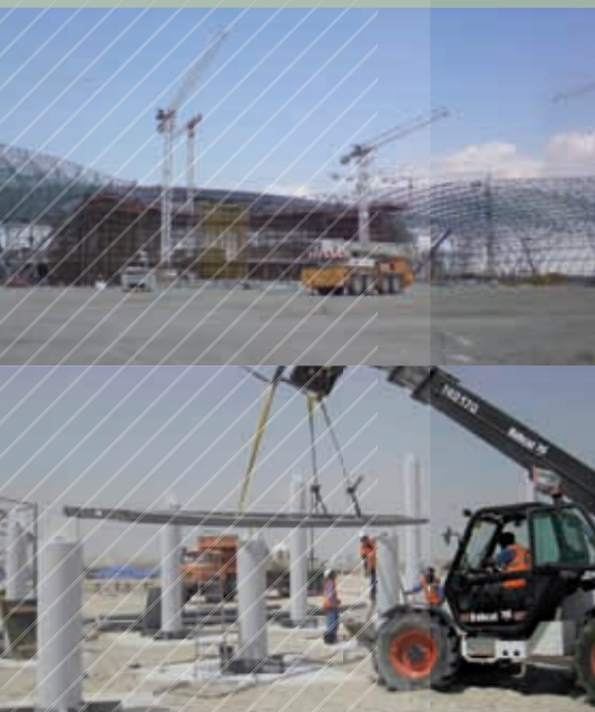
↑ Dueling Coaster, Yas Island, Abu Dhabi • (Erection of 800 tons steel structure, including control and power cable installation)
