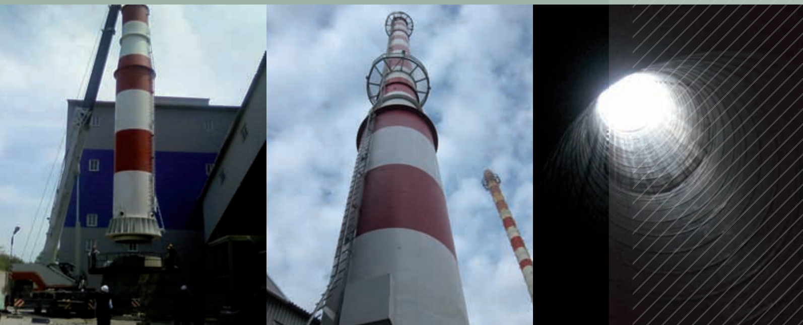
↑ 60 m stack, Glass Bottle Plant, Mineralnye Vody, Russia • (Supervision of stack erection)
